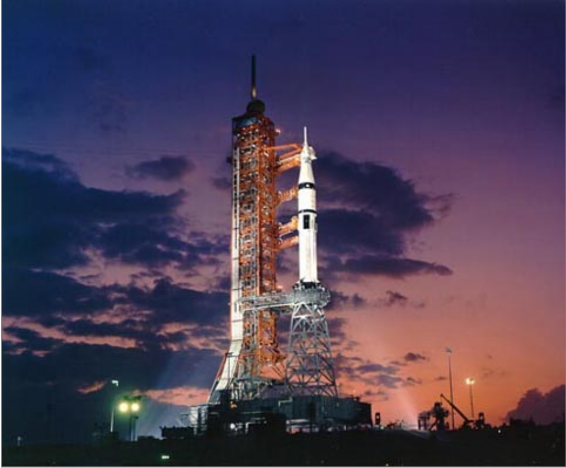
Mobile Launcher 1 was modified to accommodate the Saturn 1B vehicle for manned earth orbiting missions.
