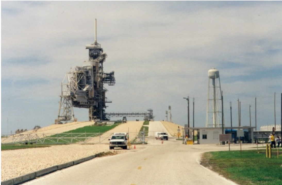
Pad 39B Shuttle Structure
